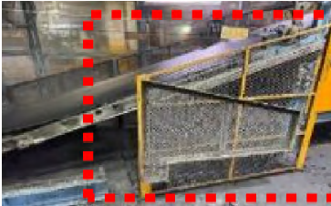
Protective railing reinstalled
