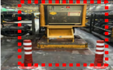
Obstructions in front of fire hydrant cleared
