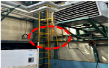
Ladder backrest cage unsecured
