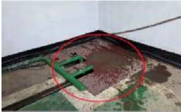
Opening cover restored
